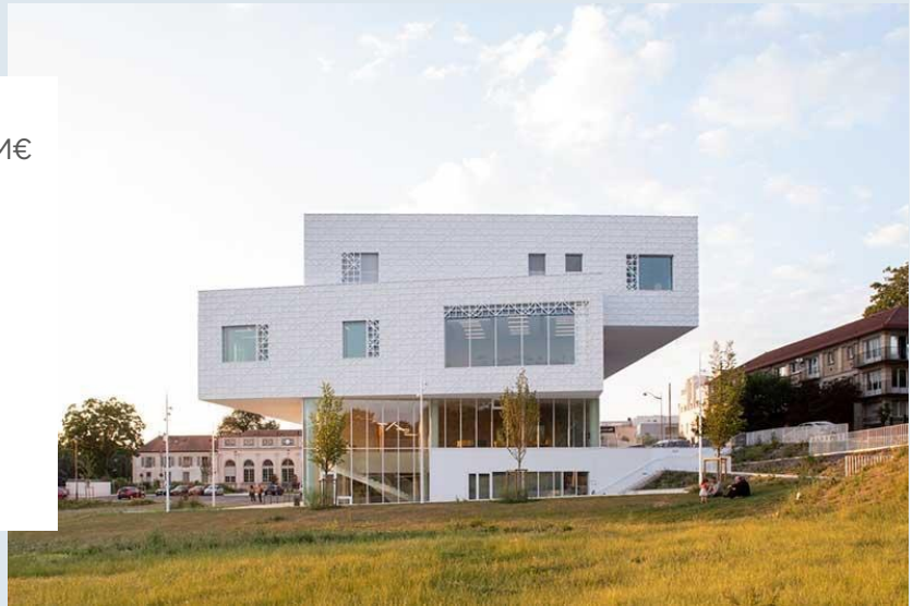
Photo credit: Gaëtan Chevrier / GPAA architectures
