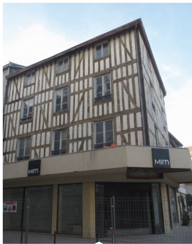
© Action Logement Services
